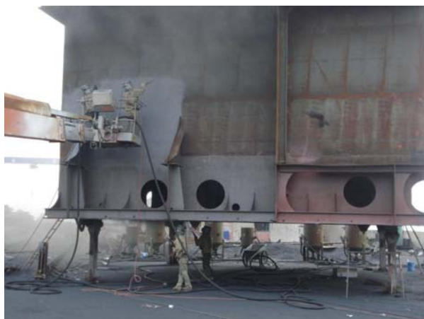
Block blasting and coating at Nantong Yahua Shipyard
