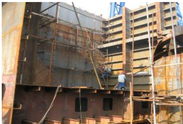
Section building at Nantong Yahua Shipyard
